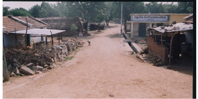
Eklaspur: Road repaired, drainage system to be finished
