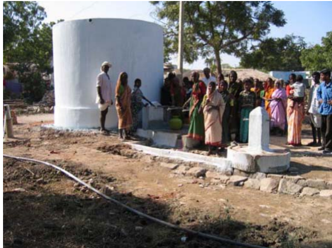
Eklaspur: Water tank
