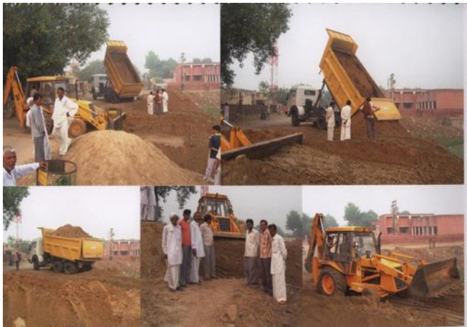
Mohabbatpur: Construction in progress (4 different scenes)
