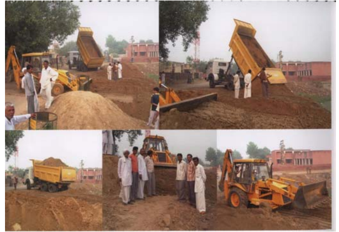
Mohabbatpur: Construction in progress 4 different scenes
