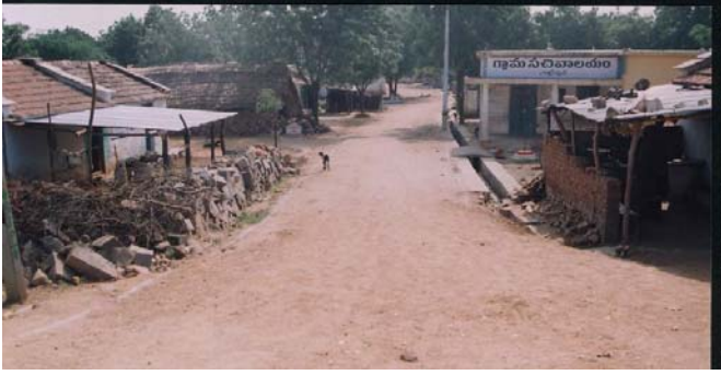
Eklaspur: Road repaired, drainage system to be finished
