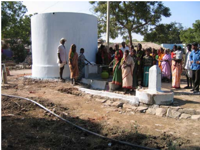
Eklaspur: Water tank
