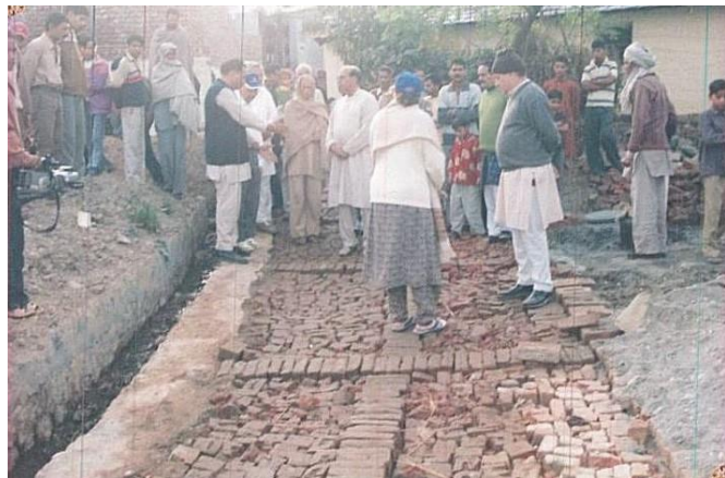
Dunera: Making base for road
