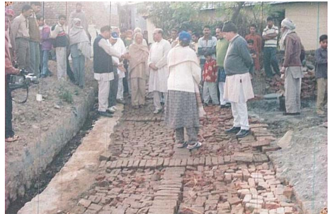
Dunera: Making base for road
