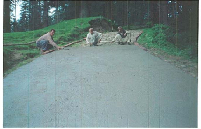
Khajjiar: Road to school being paved
